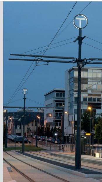
Tram - O.C.L. supports (Overhead Contact Lines)
