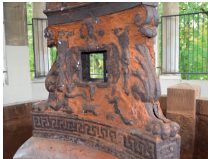
The Nancy Thermal fountain before its renovation
